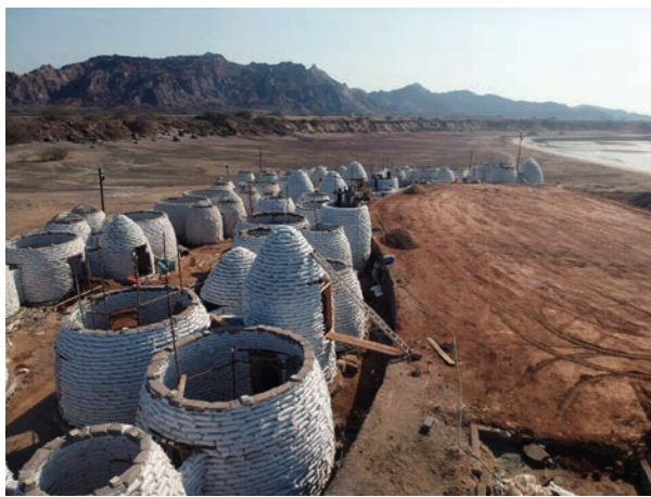
Majara Residence during construction. The domes were built using superadobe, a technique pioneered by Iranian architect Nader Khalili in the late 20th century, for which he received the Aga Khan Award for Architecture in 2004 (Sandbag Shelter). The construction method is suited to Hormuz's climate and material availability. The thick earthen walls regulate indoor temperatures, reducing reliance on artificial cooling.
