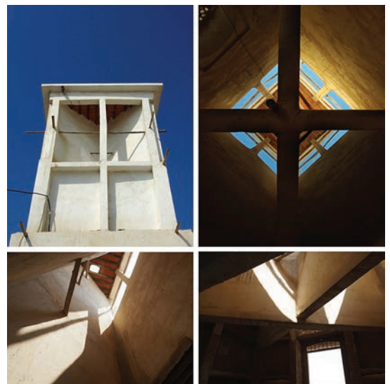
The Wind Catcher Structure
